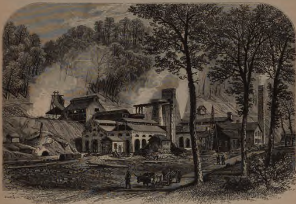
The Rockwood Iron-Furnaces—Eastern Tennessee.
